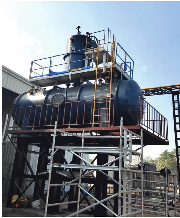
Deaerator Tank Installation (Yokohama Tyre)
