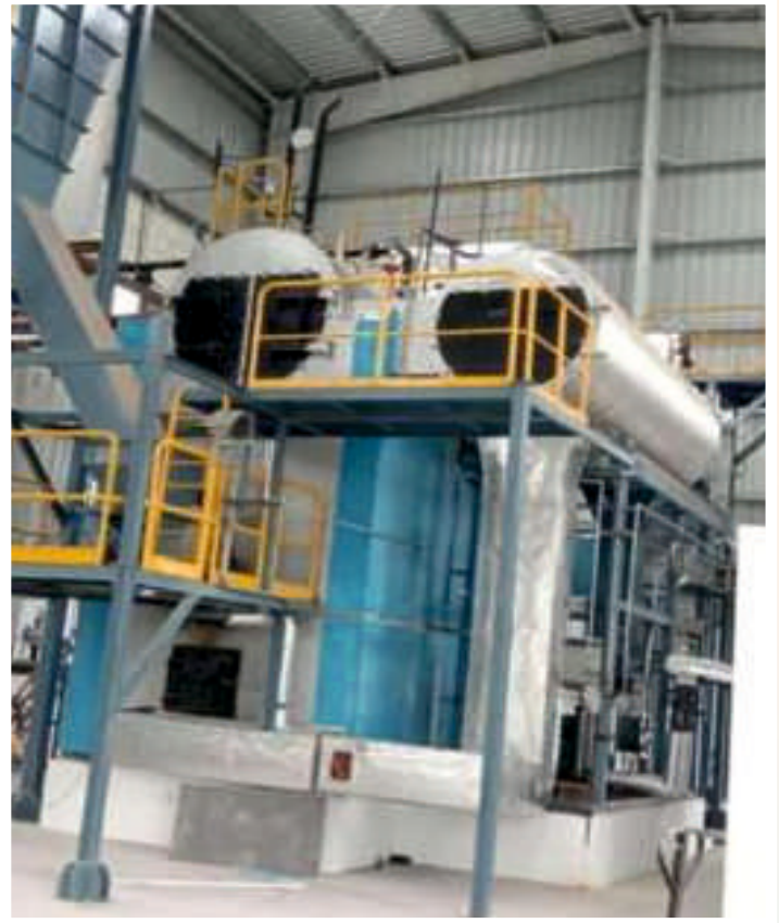
3 TPH Boiler Erection
