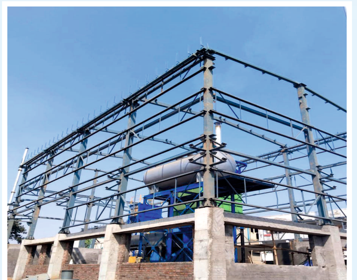
Boiler House Shed
